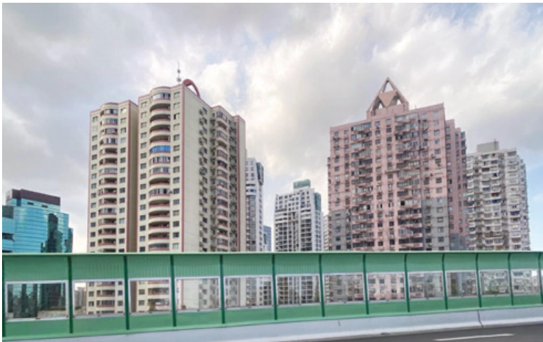
Figure 1.4 Typical residential tower blocks in Shanghai. Photo by Rui Zhong.
