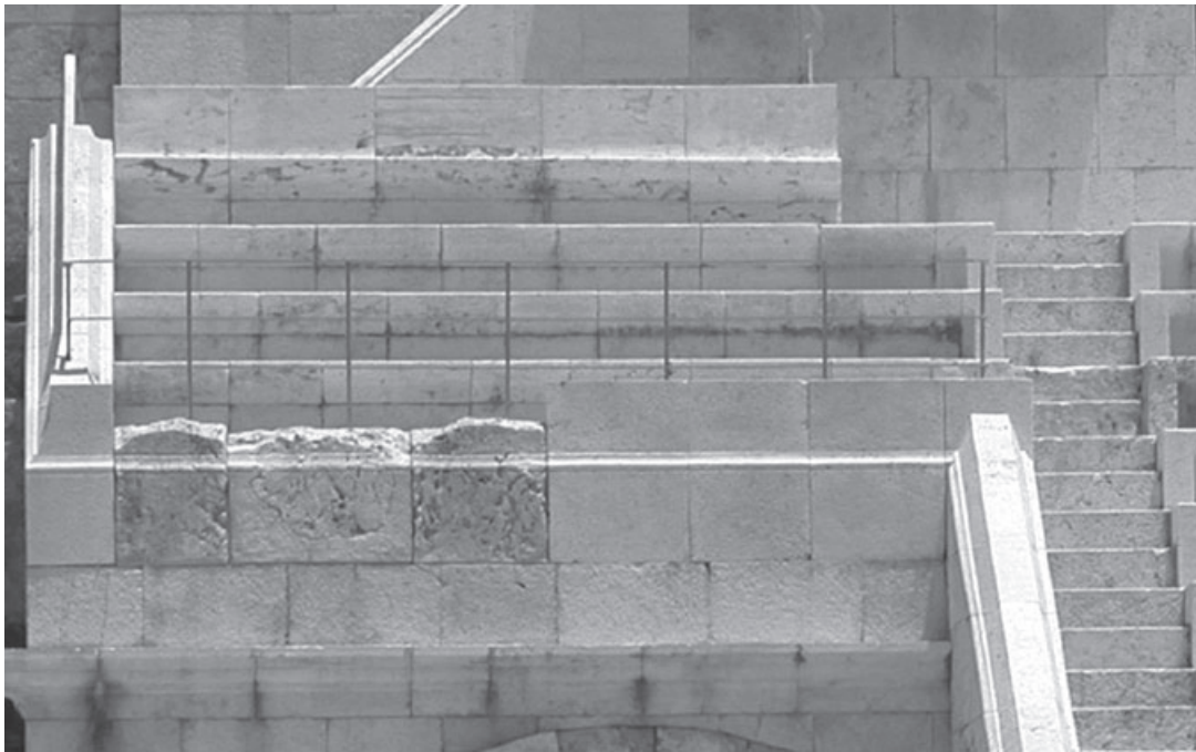
Fig. 7.25. Severan Theater: eastern tribuna after reconstruction, looking east.
