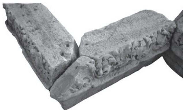
Fig. 7.10. Severan Theater: reconstruction of connection between architrave-frieze elements A6030 and A6014+A6047 over Column No. 4.
