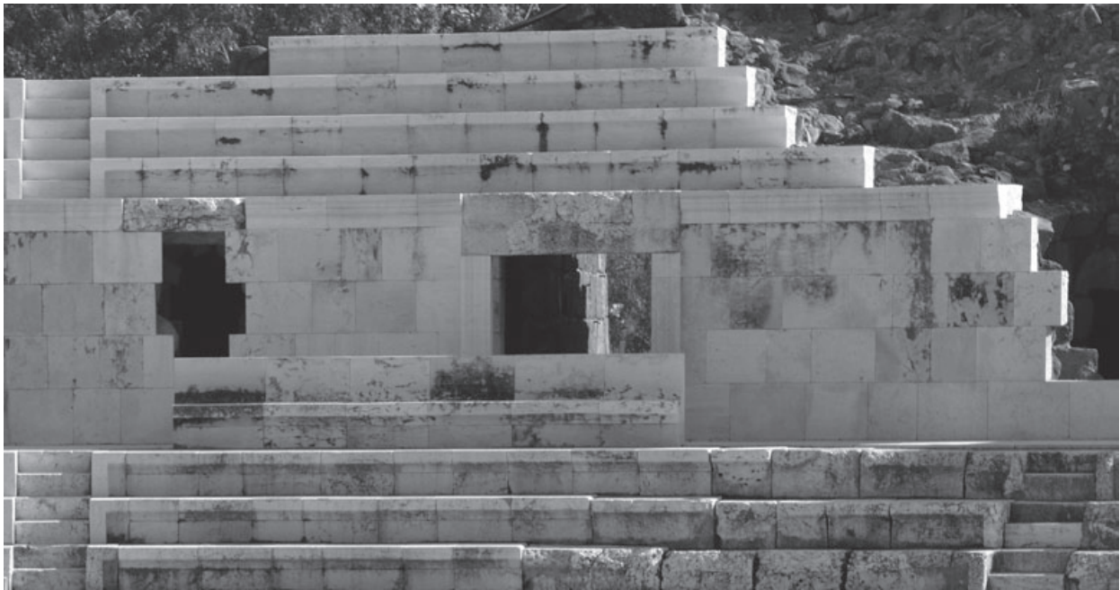
Fig. 7.28. Severan Theater: media cavea podium with vomitorium entrance and flanking staircases, looking east.
