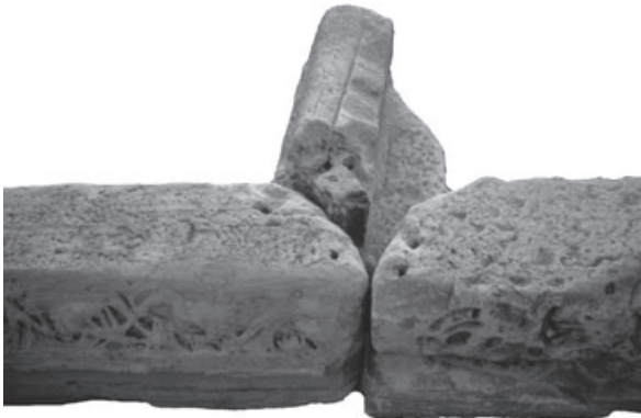
Fig. 7.12. Severan Theater: reconstruction of connection between architrave-frieze elements A6032 and A6038 with wedge member A6048 over Column No. 12.
